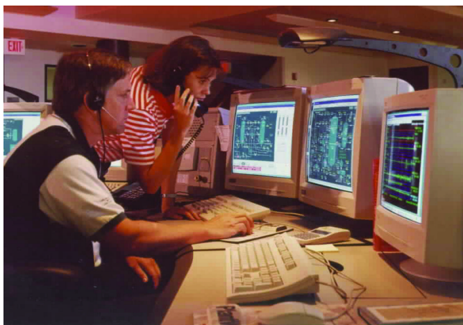
Flint Hills Resources invested $40 million in 1999 to upgrade its Corpus Christi control center.
