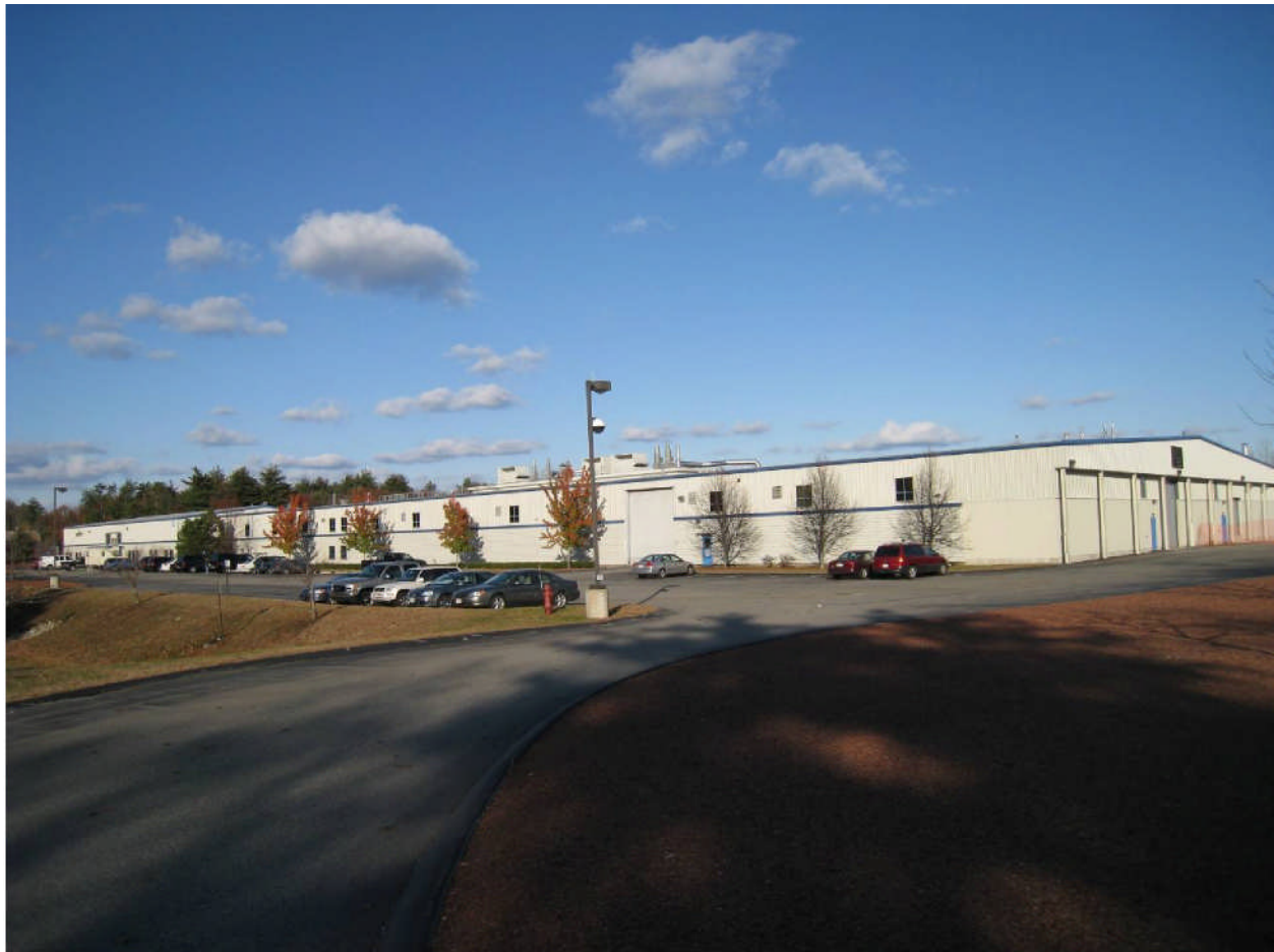
View of Building Housing New RO/NF Production Line at Koch Membrane Systems Headquarters in Wilmington, Massachusetts
