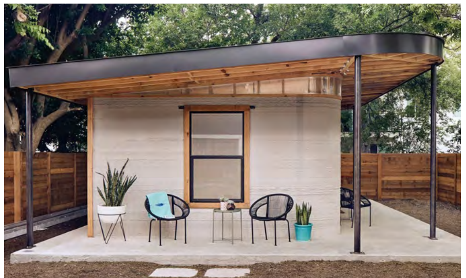
/// America's first 3D-printed house in Austin, Texas, made with ICON's innovative technology.
