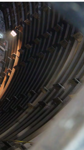
Left: New six-pass SUPERFRAC ® XT trays made by Koch-Glitsch were recently installed at FHR's Houston chemical facility. As part of this project, Koch Specialty Plant Services designed and built a special elevator that enabled the removal and replacement of old equipment in a faster, safer way.
