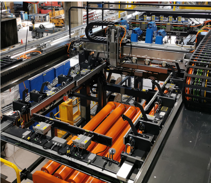
Next-generation robotic patch technology is being installed this summer.
